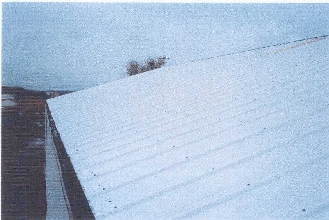
Figure 11a. 16 year old Prepainted 55% Al-Zn Coated Sheet buildings, SMP, Chromate Pretreatment
