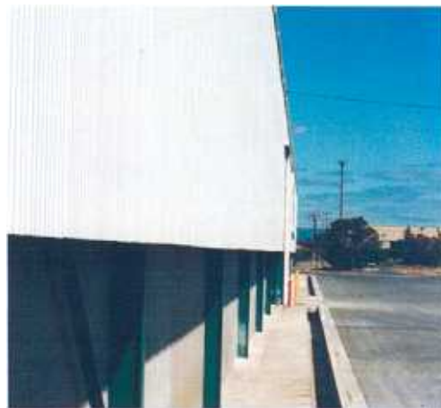
Figure 3: Example of a dwarf wall
