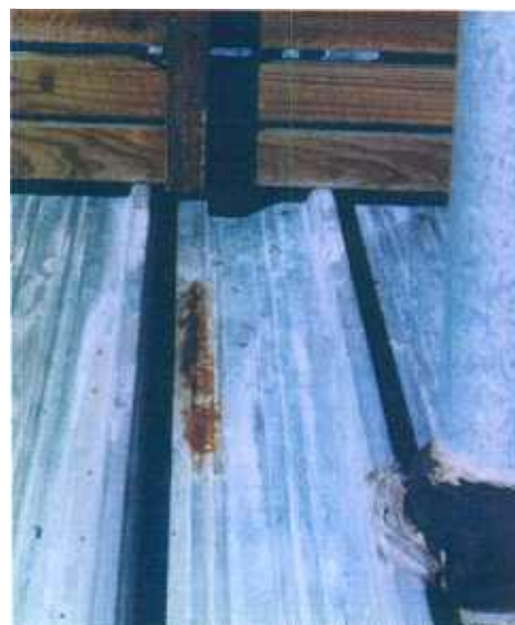
Figure 1: CCA Treated Timber Walkway
