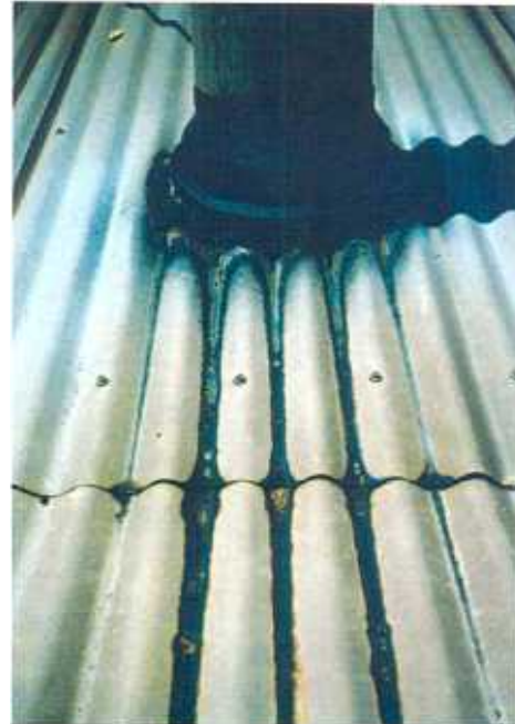
Figure 1: Flue Deposition/Corrosion.
