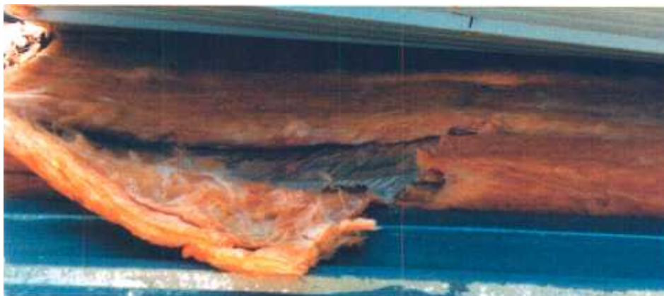
Figure 3 - Photo depicting the result of incorrect installation procedure in a tropical environment.
