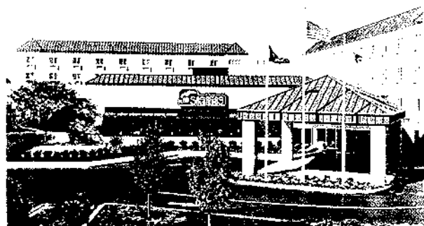
Figure 13: A pre-painted, steep slope 55% Al-Zn retro fit roof installed over a leaking non-metallic hotel roof.
