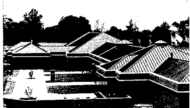
Figure 15: A steep pitched pre-painted 55% Al-Zn architectural roof on a government building.
