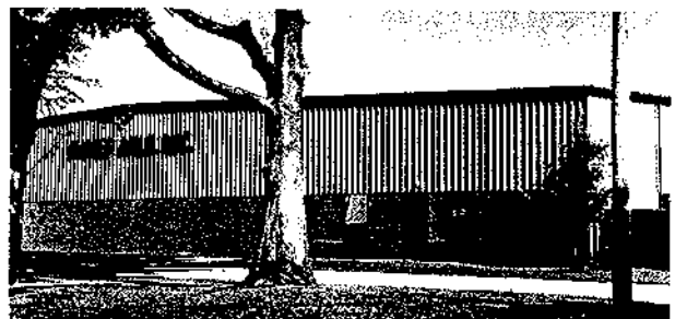
Figure 9: Typical low-rise, pre-engineered industrial building with a bare low slope 55% Al-Zn roof.
