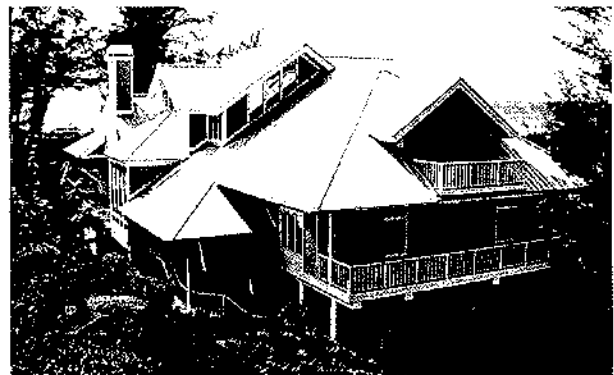
Figure 16: A steep pitched pre-painted 55% Al-Zn residential roof on a home near the ocean.
