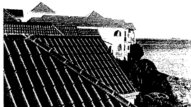
Figure 17: A pre-painted, tile facsimile 55% Al-Zn roof on a condominium near the ocean.
