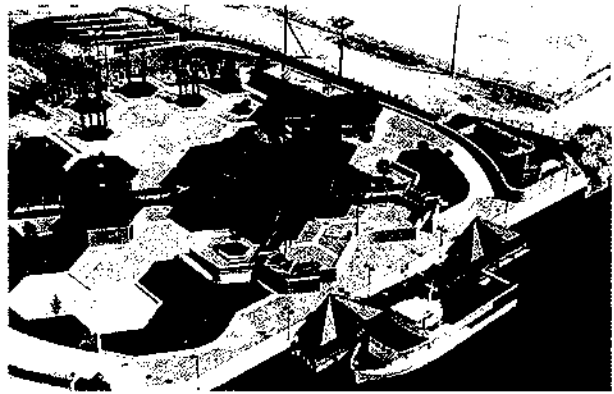
Figure 14: A steep slope, complex shaped, pre-painted 55% Al-Zn roof on a visitors centre.
